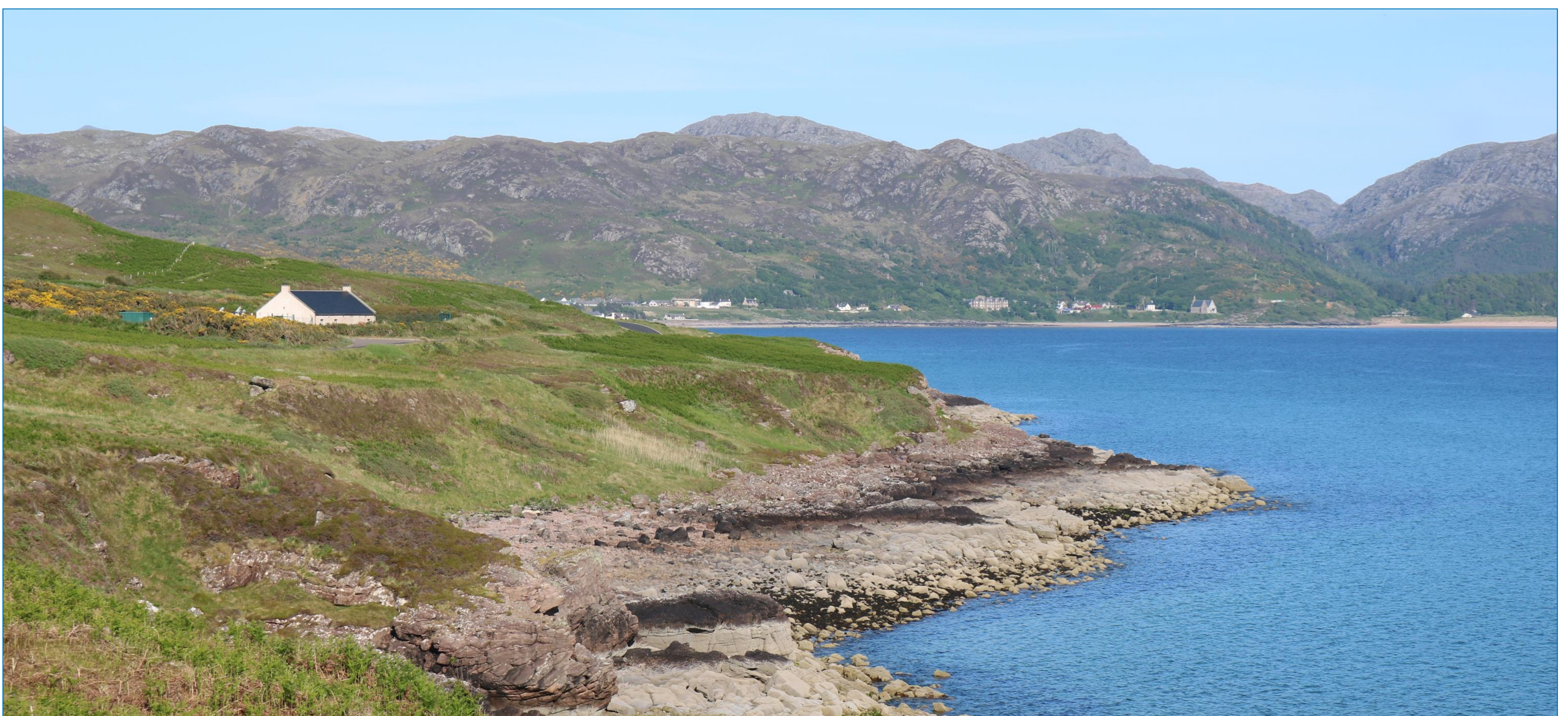
Gairloch Waste Water Treatment Works, viewed from the West
