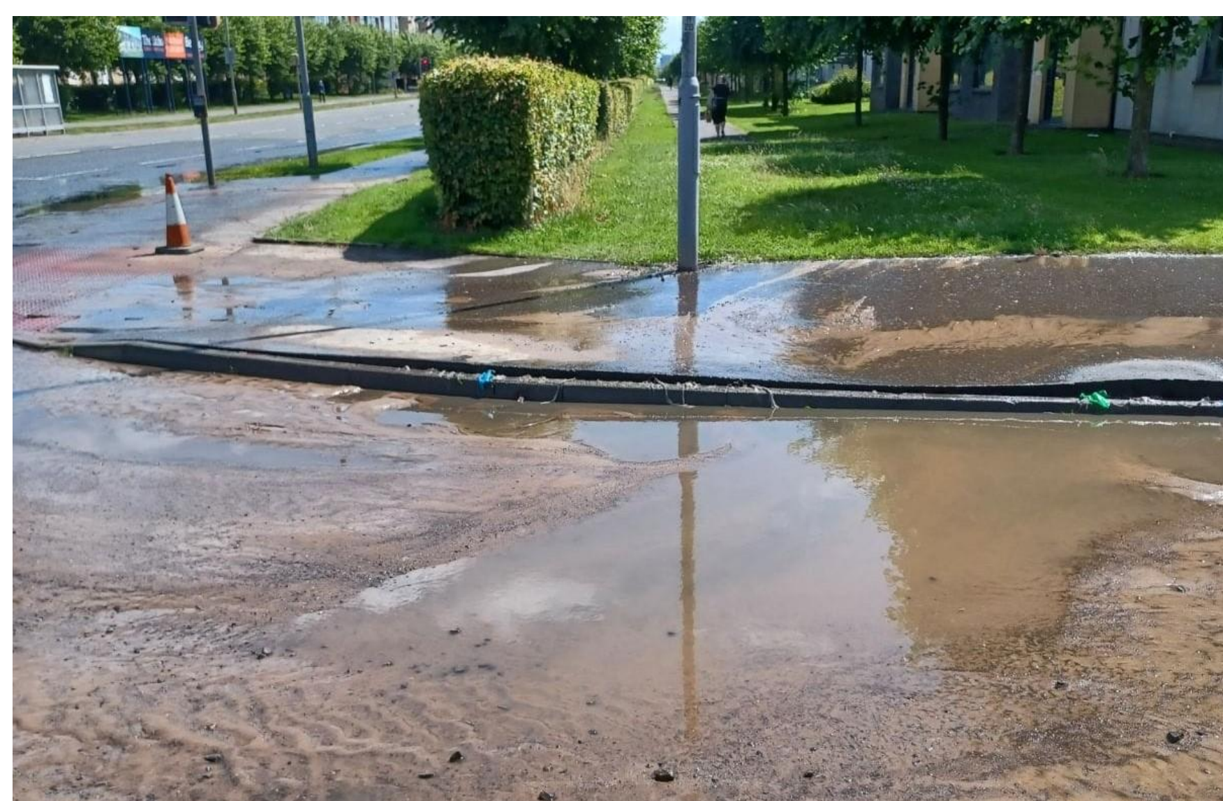
Burst incident on Kings Inch Road 2023
