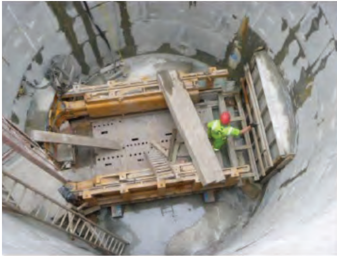
Construction of tunnel drive shaft
