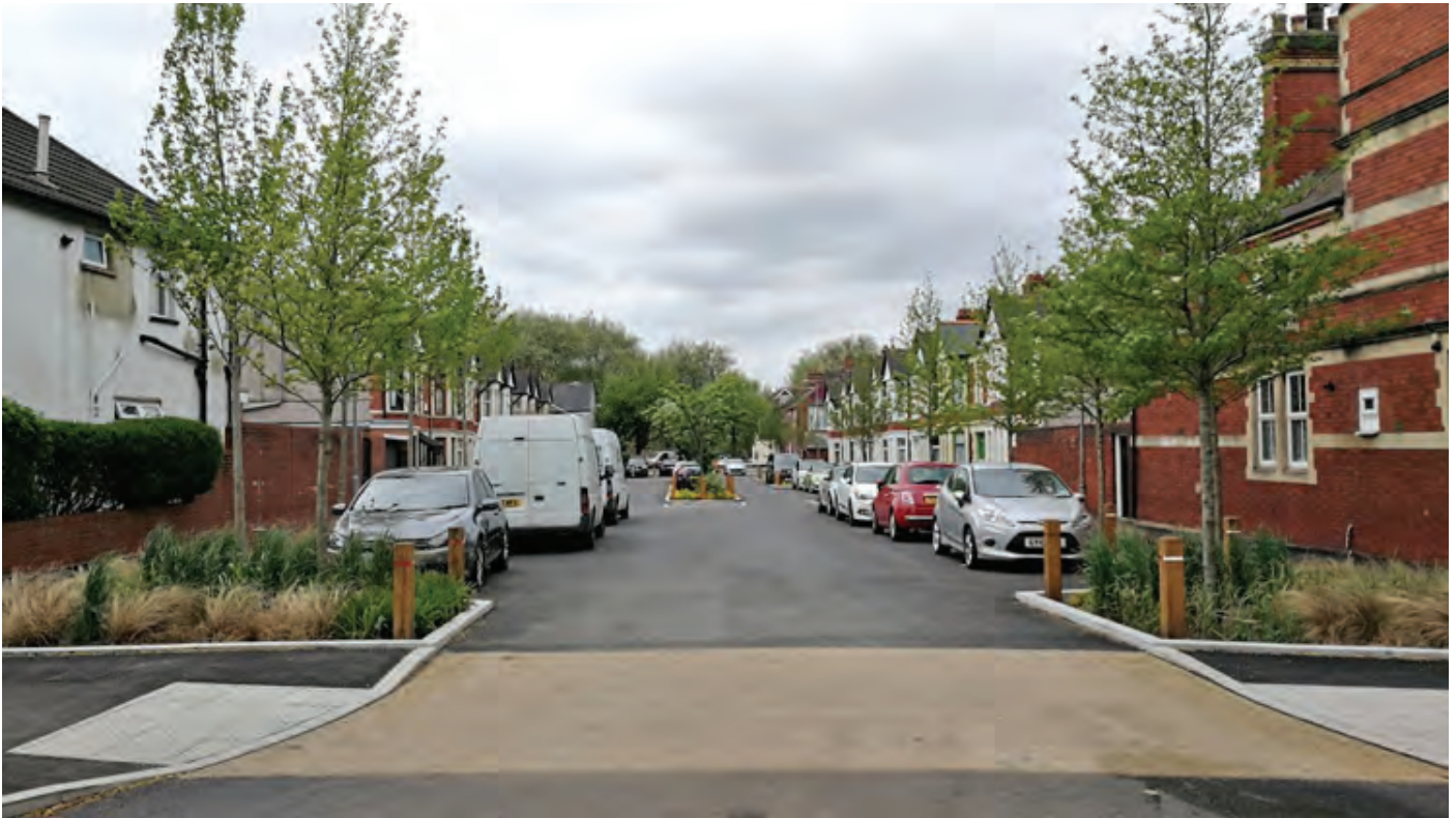
Retrofit Highway Raingardens delivered by the Greener Grangetown Project
