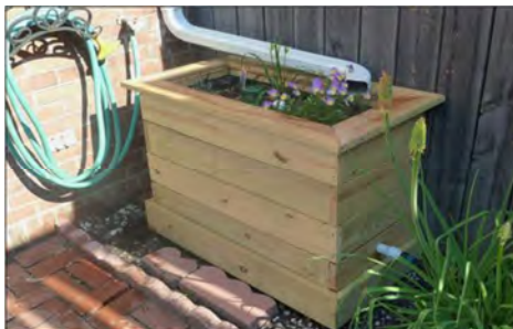
Disconnecting downpipes into planters or water butts
