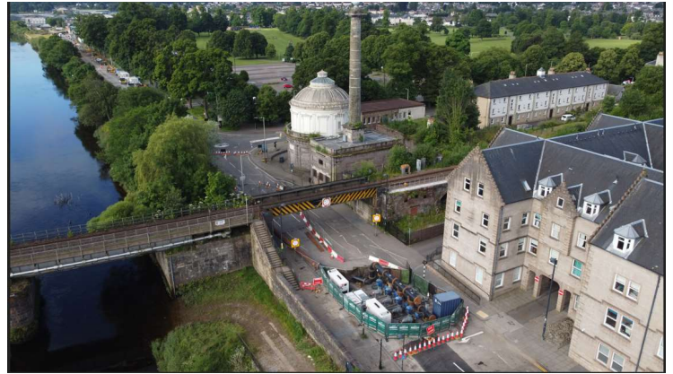
Image: Drone footage of over pumping set up.
