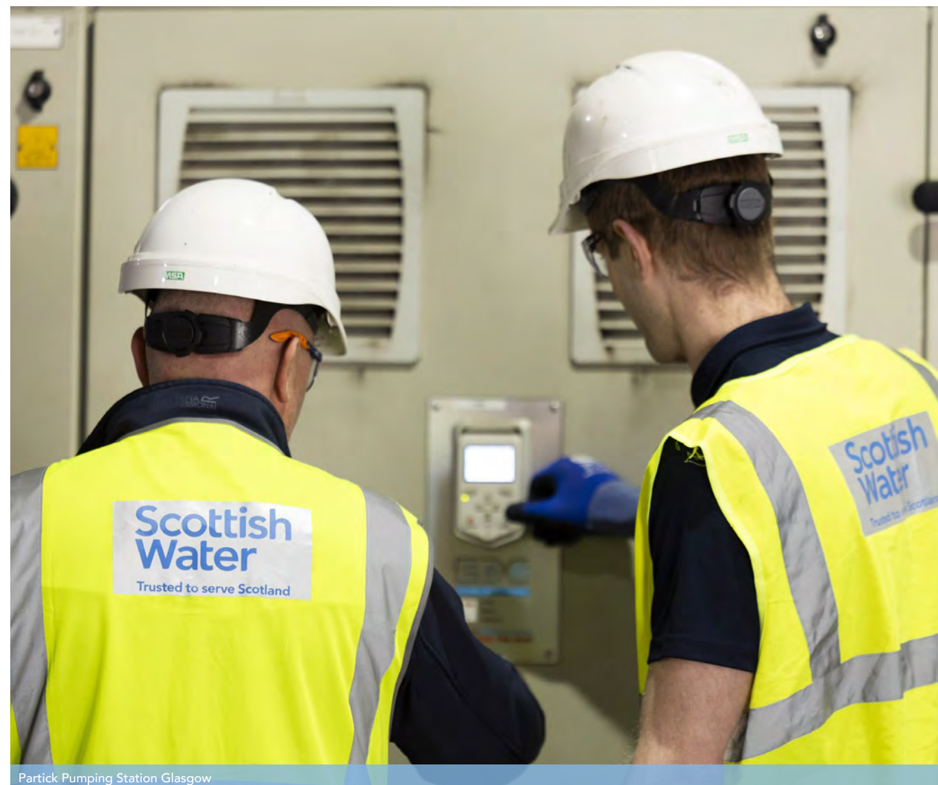
Partick Pumping Station Glasgow
